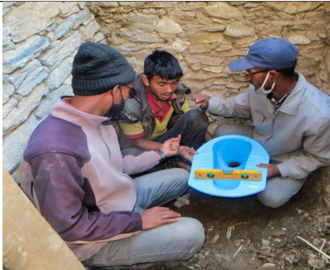
PIC.92. Two Pere project staff teach how to fix the toilet pan in new constructed PL.
