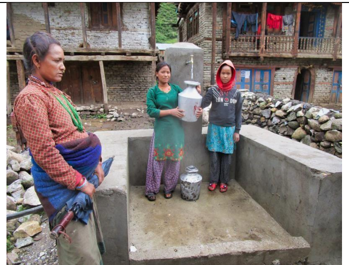
Pic. 33: A finished tap stand in Pere village providing now 2 hours in the morning and 3 hours in the evening water for the Pere families. Each family has to walk now only 1-3 minutes to fetch sufficient, clean, drinking water
