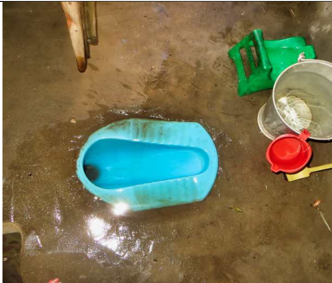
PIC.94. Inside view of a newly built Pit Latrine in Pere village.
