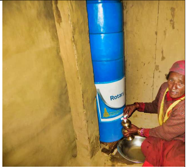
PIC.139. A Pere woman uses clean drinking water from the newly installed SSWF.
