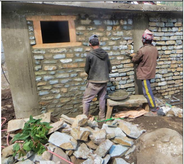
PIC.111. The skilled labors are giving finishing touch to newly constructed SHWBC cabins.
