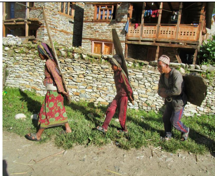
Pic. 43: The use of wood is as much as possible reduced. Here a family carries slates to cover the prepared PL septic tank
