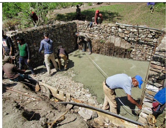
Pic. 20: Measuring and cementing the floor of the 25m 3 storage water tank under guidance of the RIDS-Nepal staff Bam Bahadur, to assure the storage tank size is sufficient
