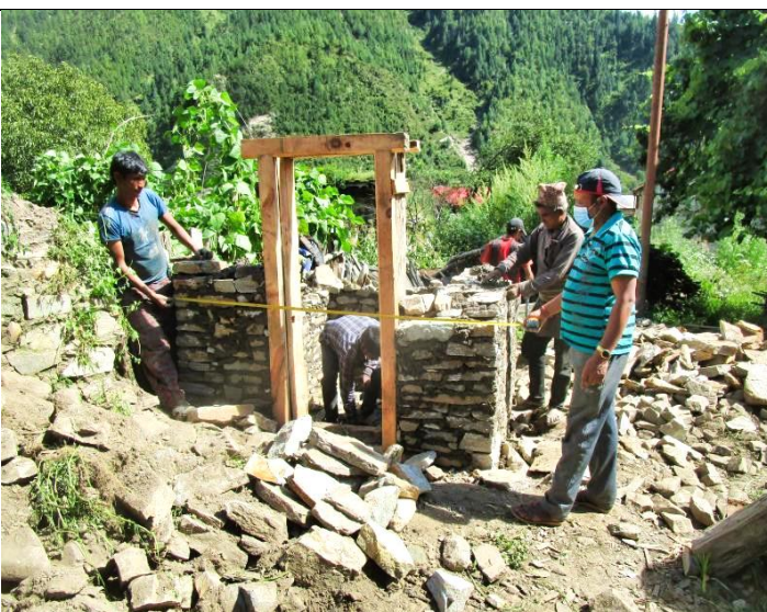
Pic. 52: RIDS-Nepal staff Mansingh checks with the measuring tape if the PL is correctly built and advises accordingly
