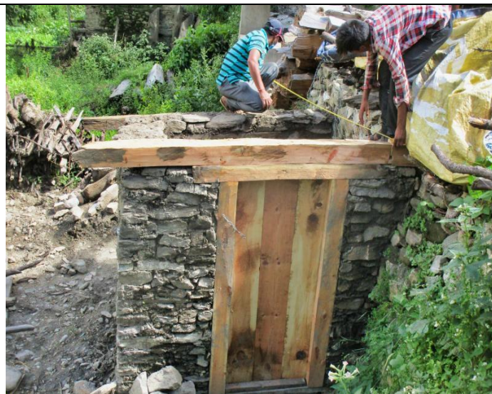
Pic. 55: The length of the PL roof is measured to assure that the three galvanized tin roofs fit as designed on the PL roof
