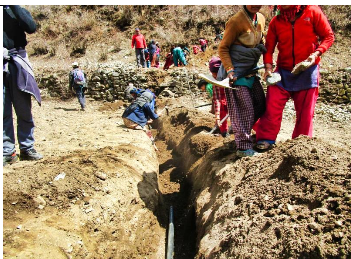
Pic. 9: The installed HDP water pipe is covered with stones and mud so that their position does not shift. This protects it against unforeseen damage; be it through agricultural work, freezing in winter or future digging. Since the water pipe runs sufficiently deep underground, the farmers can cultivate the fields above as normal
