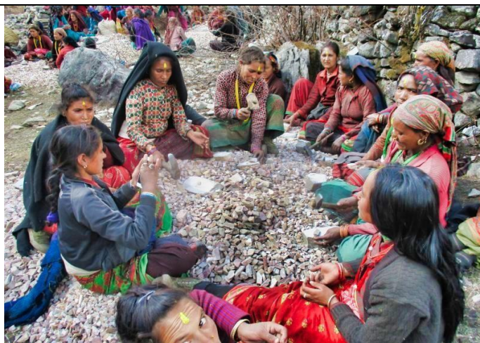
Pic. 15: Women smash big stones with the hammer into pebbles to be mixed with sand and cement for mortar
