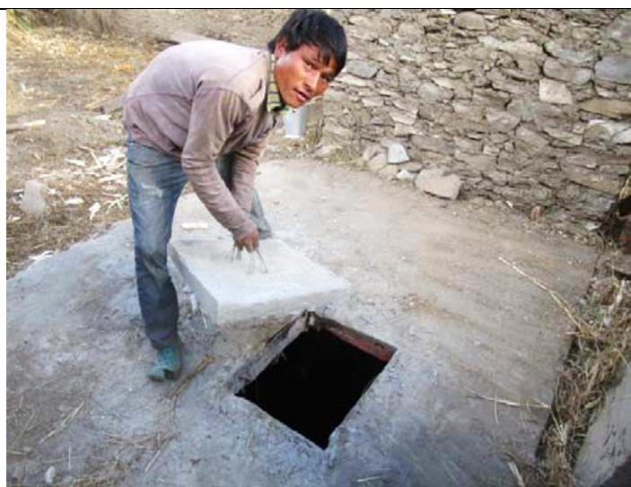
Pic. 64: A newly constructed septic tank for the family pit latrine which can be used for approximately 8 years before it needs to be emptied for re-use
