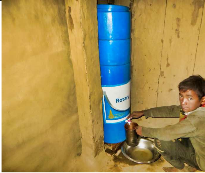
PIC.144. A Pere boy uses clean drinking water from the newly installed SSWF.
