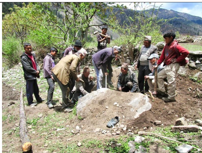
Pic. 16: One of many big boulders, in the way of the source intake, has to be smashed by hammer and removed by hand
