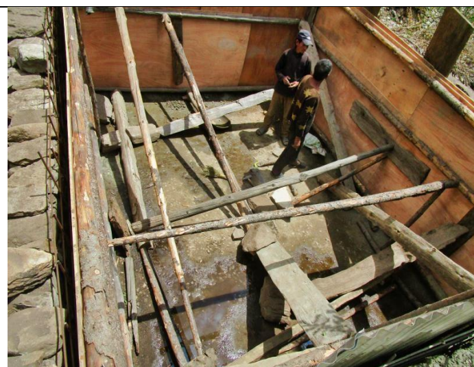
Pic. 21: Metal rods, all prepared and cut to size by hand, are used to reinforce the storage water tank cement walls to avoid any leakage and for maximum strength and durability
