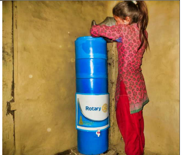
PIC.135. A Pere young girl is filling her newly installed SSWF in her family's home to store and filter the drinking water from the tap stands in the village.
