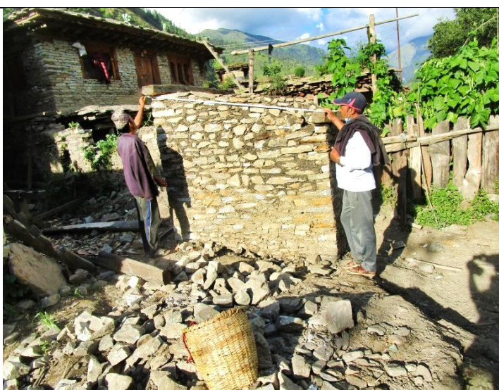
Pic. 56: The length of the PL roof is measured to assure that the three galvanized tin roofs fit as designed on the PL roof
