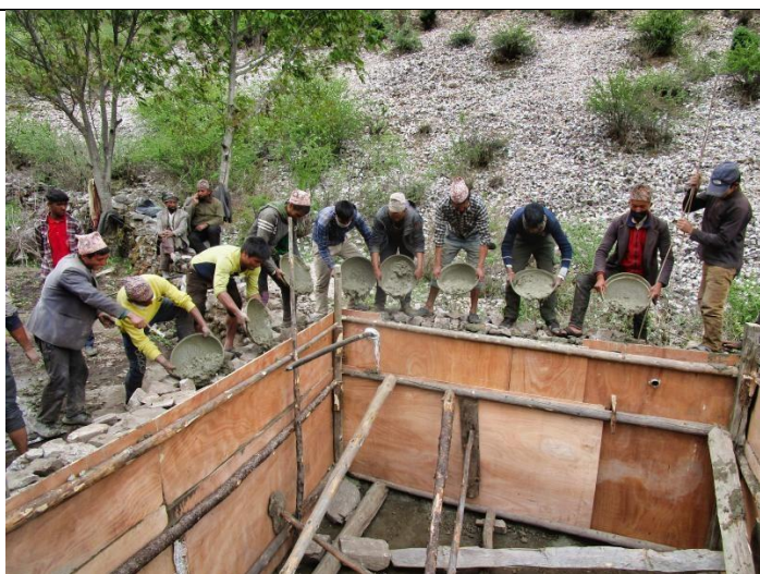
Pic. 22: All the cement is prepared with the collected sand from the river (Pic. 4) and prepared pebbles (Pic. 5) under the guidance and supervision of the RIDS-Nepal staff. The prepared cement is carried and dropped into place by hand
