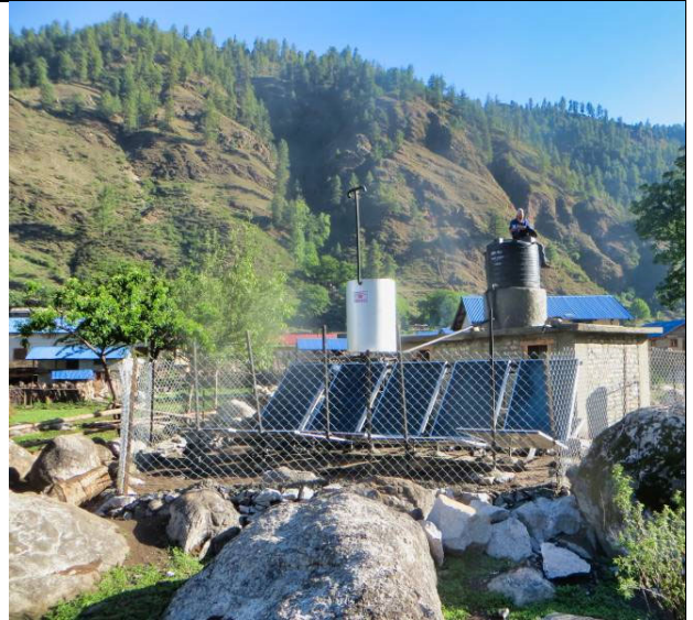
PIC.117. A fully completed SHWBC in Pere village.
