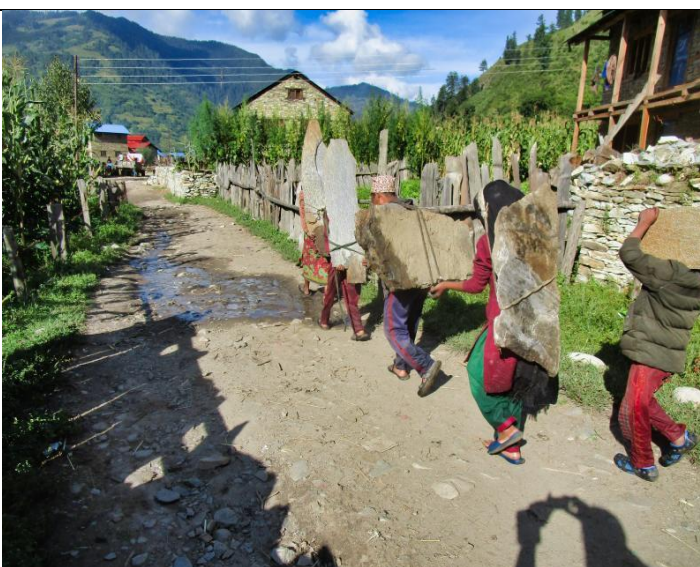
Pic. 44: Slate plates are prepared in a nearby quarry and carried home to cover the PL septic tank
