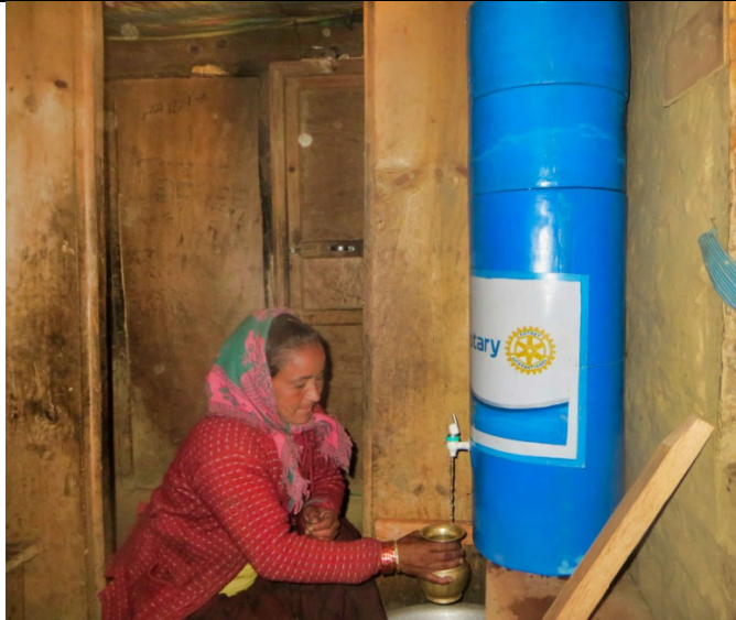
PIC.140. A Pere woman uses clean drinking water from the newly installed SSWF.
