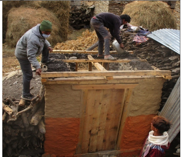
PIC.91. A family PL stone house is built with ready to cover with tin roof.
