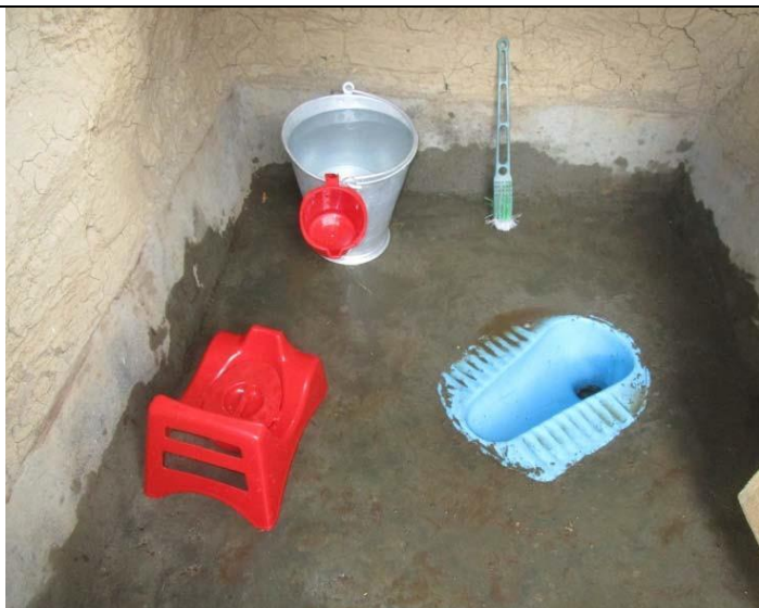
Pic. 66: A fully completed pit in picture
