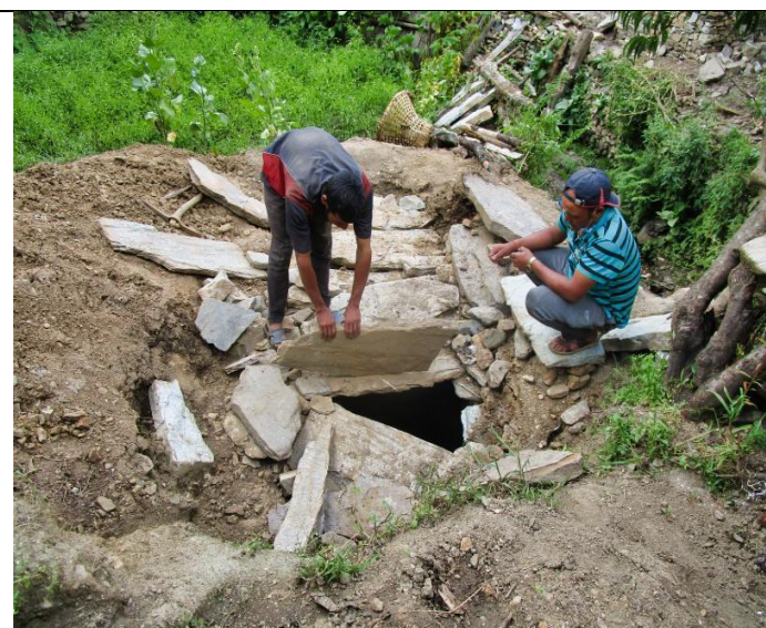
Pic. 45: With the prepared slate plates the built PL septic tank is covered. Additionally, mud is laid on top of the slate plates
