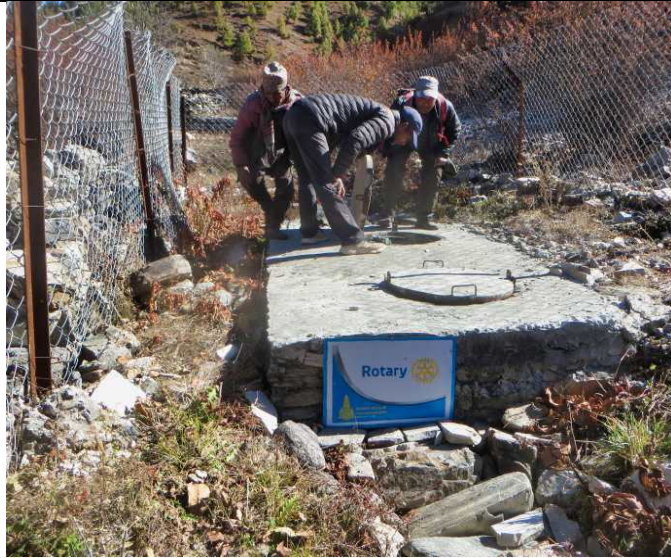
PIC.162. Ongoing inspection and cleaning of the 25m3 seized DWS (Drinking water system) water storage tank by Pere project staff and local trained maintenance people.
