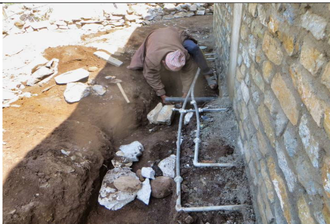
PIC.112. The skilled labors are installing pipelines for both cold and hot water systems in Pere.
