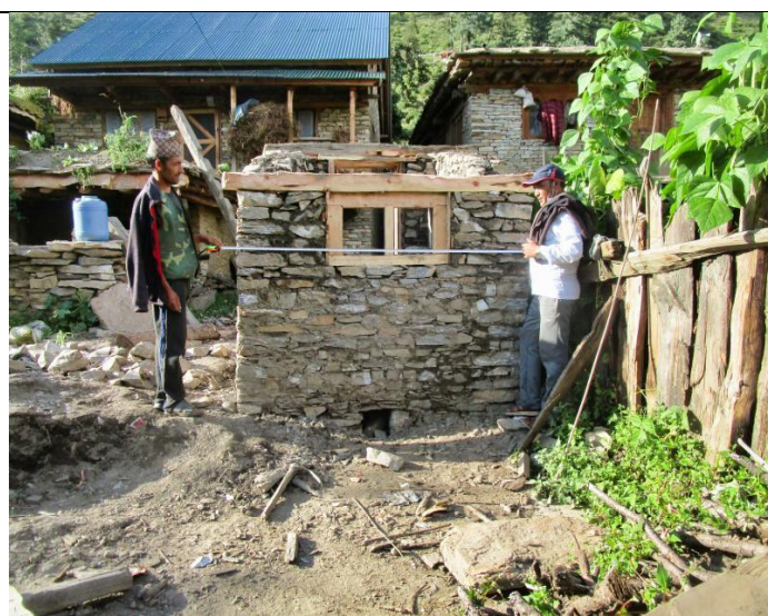
Pic. 57: The width of the PL is measured to assure that the insides dimensions are kept as per designed RIDS PL standard
