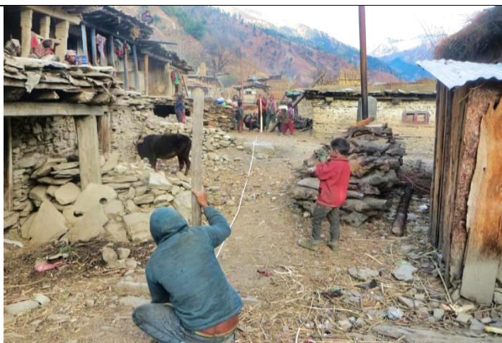
Pic. 3: The water pipes in the village are laid in such a way that all residents can get their daily water for family and animals from one of the 15 tap stands within 1-2 minutes walking distance
