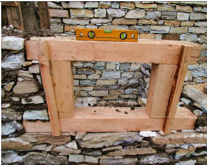
Pic. 50: The air ventilation PL window is leveled out with the spirit level before it is integrated into the PL stone wall
