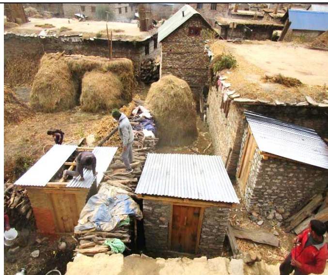
Pic. 61: A Pere family is roofing his toilet
