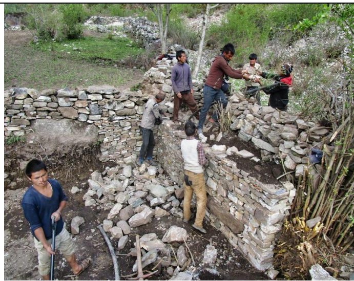
Pic. 19: Preparing of and start building the 25m 3 sized drinking water storage tank above Pere village, collecting the source water flowing constantly into it safely
