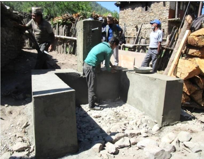
Pic. 32: One of the Pere village tap stands gets the finish top layer of cement which is a 1:1 cement-sand mixture to create a smooth and water proof surface, providing the tap stands' walls with a long-lasting protective surface
