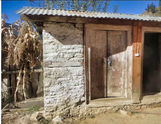
PIC.98. A Pit Latrine in Pere which is in use since July 2020.
