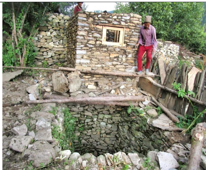
Pic. 59: A family PL stone house is built with the ready to cover septic tank to collect the liquid and solid effluents
