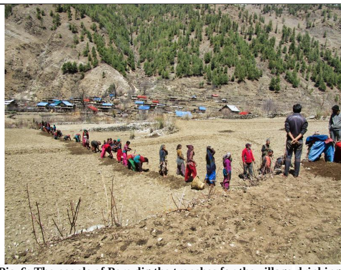
Pic. 6: The people of Pere dig the trenches for the village drinking water system. One person digs every ~ 2 meters so that the entire water pipeline can be laid in the shortest possible time. Every family sends at least one person every day to work on the new village drinking water system
