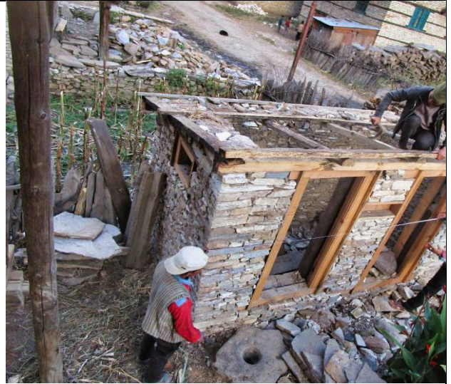
PIC.89. 2 PLs are built together due to lack of land. Length of the PL roof is measured to assure that the three galvanized tin roofs fit as designed on the PL roof.
