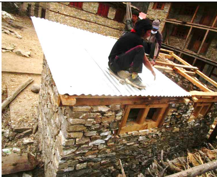
Pic. 60: A Pere family is roofing his toilet
