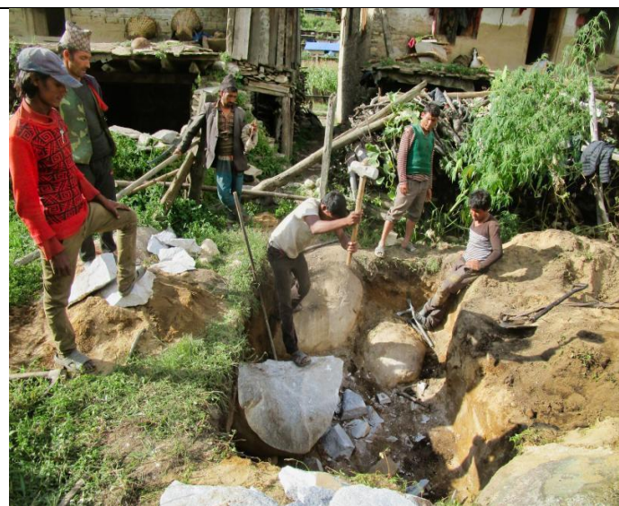
Pic. 41: Often huge boulders prolong the work to get the septic tank for the PL dug out according the required measurements
