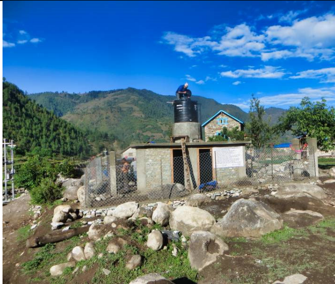
PIC.116. Installation of SHWBC are ongoing.
