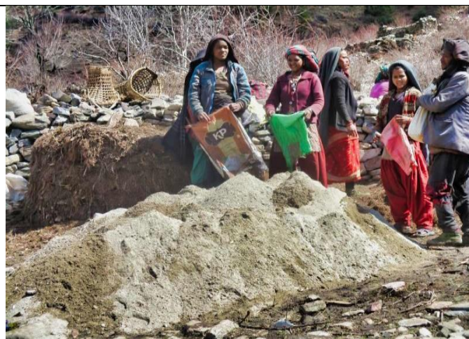
Pic. 4: The sand required for all cement work is collected from the local river bed. This is sieved so that the correct sand grain is achieved
