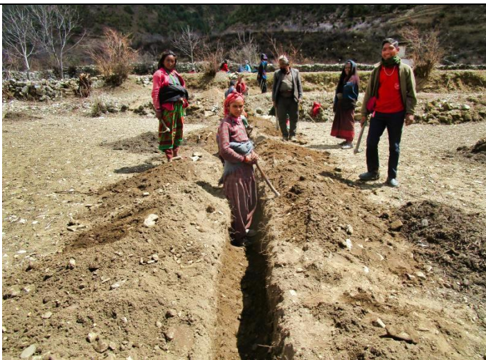
Pic. 7: The trenches are 50-60cm deep and 50 cm wide so that the water in the pipes never freezes, even in winter. People from the PIC team trained by RIDS-Nepal, check compliance with the prescribed depth
