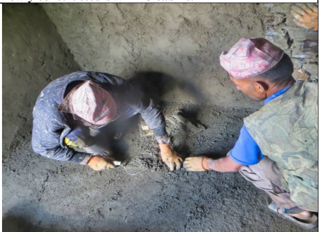
PIC.113. The skilled labors are plastering the walls and floors of SHWBC in Pere.
