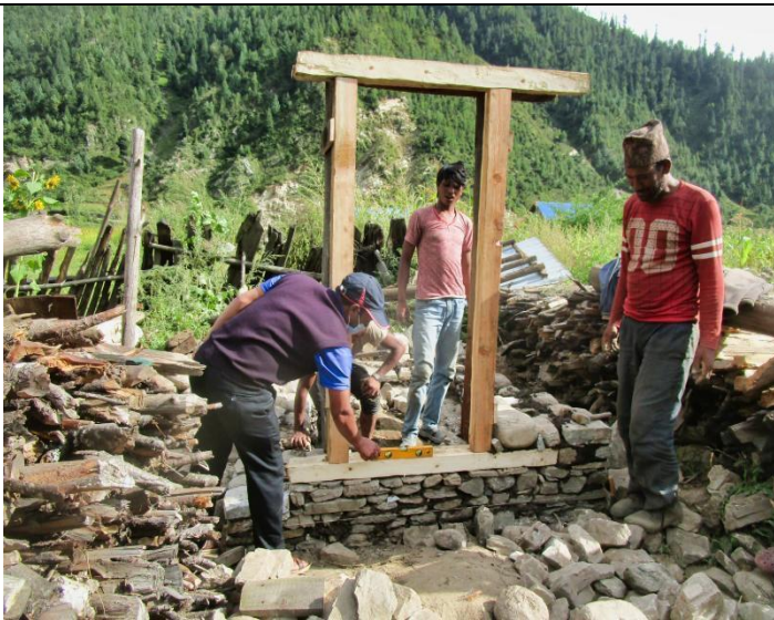
Pic. 48: RIDS-Nepal staff assure that the PL door foundation is leveled before building the stone wall around it
