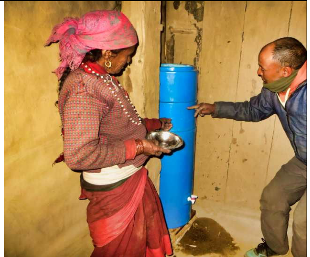
PIC.131. Mansingh provides onsite training support in the installation of a SSWF.
