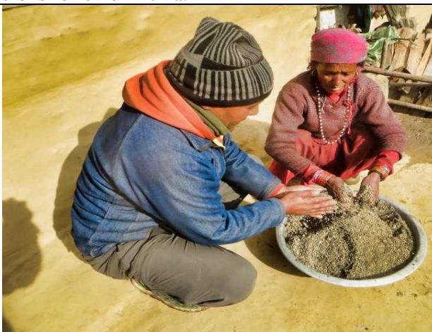
PIC.125. Mansingh (RIDS staff) teaches how to prepare/wash the sand for the SSWF.
