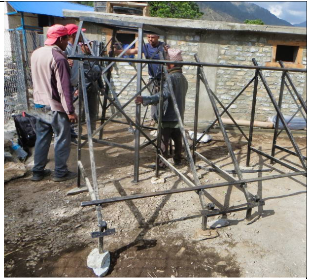
PIC.115. The skilled labors have set up metal frame to installed SHWBC system.
