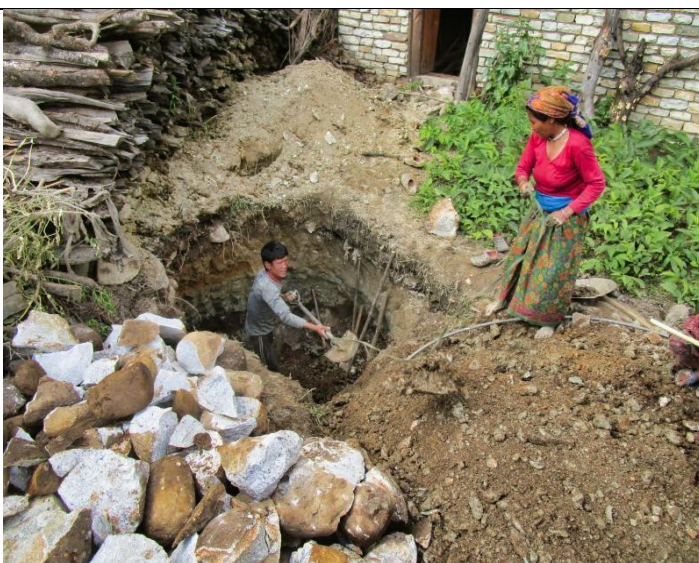
Pic. 40: One of the major tasks for each family is the digging out of the septic tank for the PL, often a very hard job
