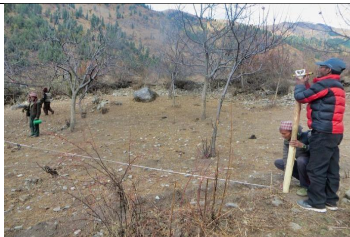
Pic. 2: Plans as well as precise material and equipment lists are drawn up for the laying of the high-density polyethylene (HDP) water pipes. The total length of the water pipes (from the source to Pere and the distribution to the 15 taps in the village) is ~ 3 km
