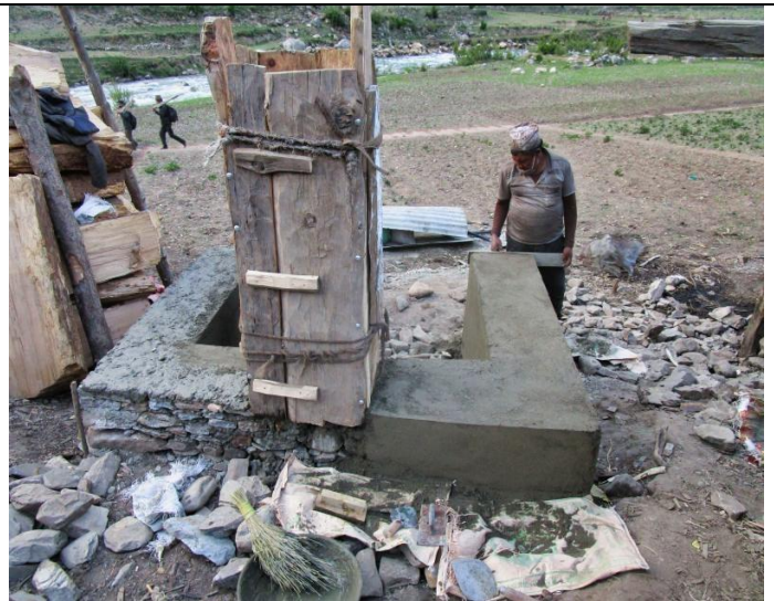
Pic. 31: The local people collect and prepare all the needed stones to build each of the 15 tap stands, before the walls are cemented for the needed rigidity of the tap stand structure
