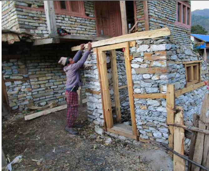
PIC.90. A family PL stone house is being built.
