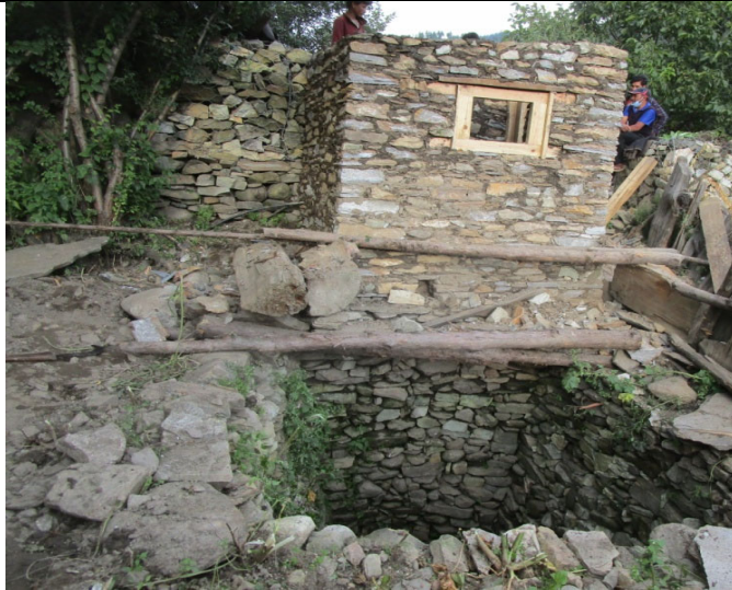
PIC.88. A family PL (Pit Latrine) stone house is being built with the ready to cover septic tank to collect the liquid and solid effluents.
