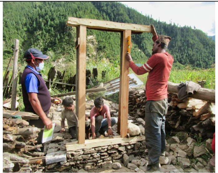
Pic. 49: RIDS-Nepal staff teaching the family how to assure their PL is built straight before building the PL stone walls
