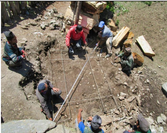
Pic. 30: RIDS-Nepal staff Bam Bahadur teaches the local people how to set up a tap stand foundation, by lining out the main stone walls and measuring that all is at correct angles
