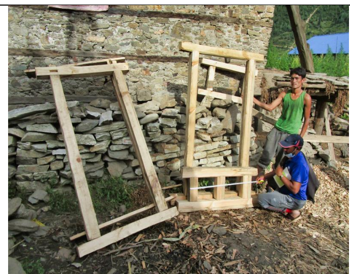
Pic. 47: Main Pit Latrine door frame, door and a small window to ventilate the Pit Latrine are made by each family under guidance and supervision of RIDS-Nepal's staff
