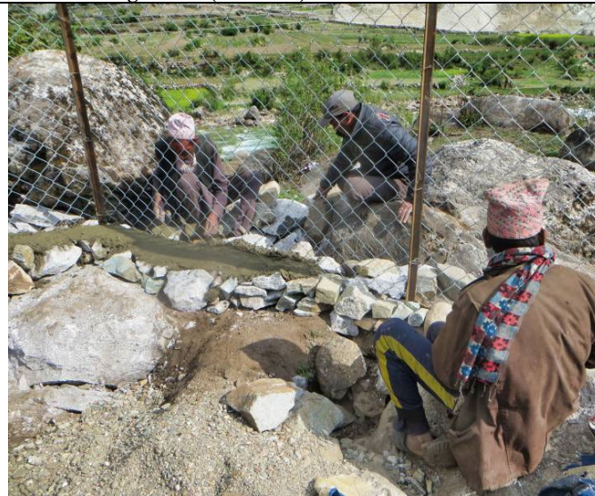
PIC.110. Pere communities are working on SHWBC.
