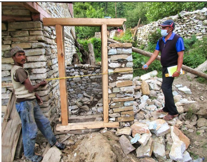
Pic. 54: Another family which builds their ne PL attached to the home as they do not have sufficient land but want the Pit Latrine
