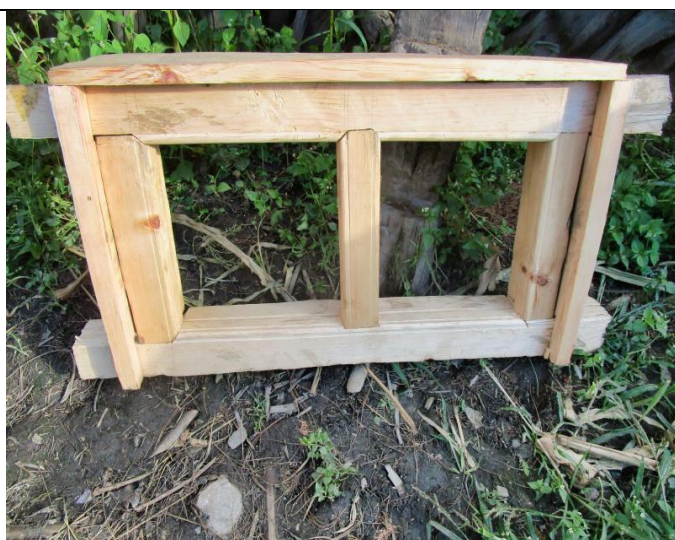
Pic. 46: A window for the Pit Latrine is produced to enable some air ventilation. The skill training for the families with no carpentry skills is provide by RIDS-Nepal
