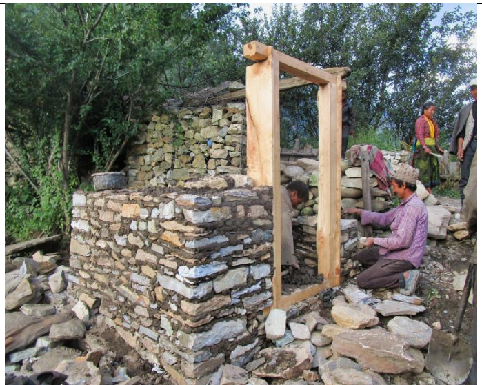
Pic. 51: Once all is leveled out and according to the RIDS- Nepal design and sizes the PL stone walls are built
