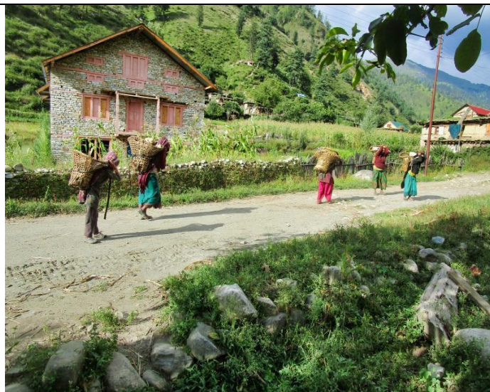
Pic. 37: Mostly it is the Pere women who carry all the stones for the Pit Latrine house structure and septic tank from the nearby quarry
