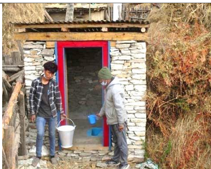
Pic. 65: A newly built and fully completed pit latrine already in use by the family who owns it. RIDS staff Bam Bahadur inspects the pit latrine if it is maintained correctly and hygienically
